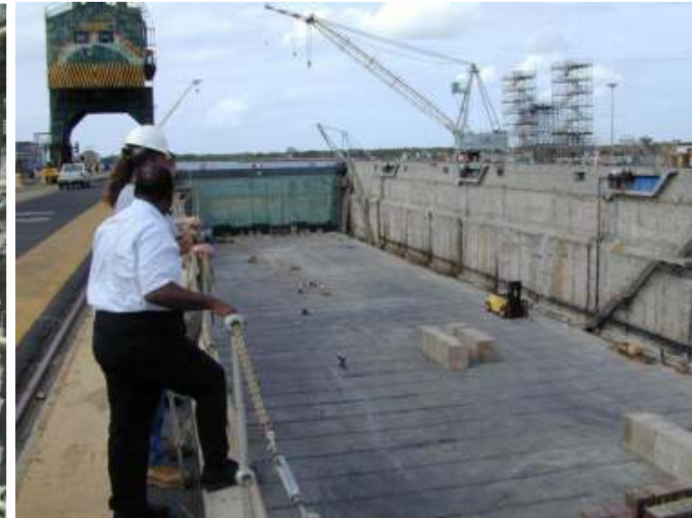
Dry Dock rehabilitation - Pearl Harbor
