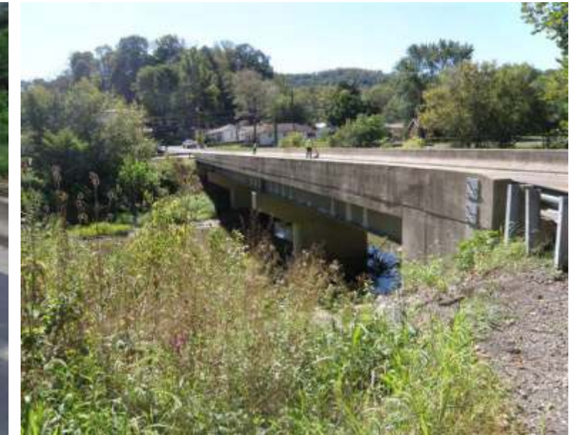
1st Bridge with FRP Rebar
