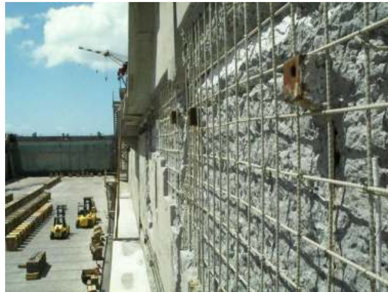
2001- Dry Dock rehabilitation- Pearl Harbor - Multiple Dry Docks
